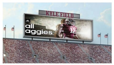
hen the gates open at Kyle Field this fall, fans will be treated to the largest video board in college football. The new video board, built by Daktronics, will measure 47-feet tall by 163-feet wide (7,661 square-feet), almost twice the size of the previous video board. It will also be the first display at the college level to feature 1080 resolution.
